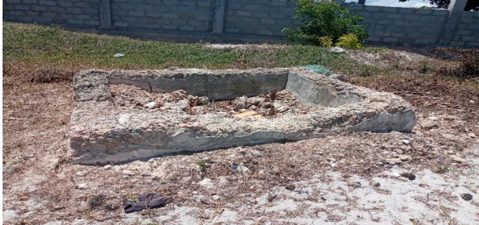
Photo 4.5: Deterioration of graves at Mbuamaji in Dar Es Salaam, November, 2021
