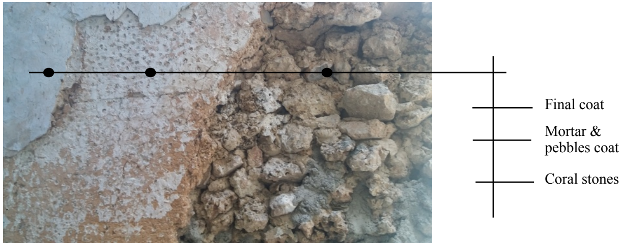
Fig. 8: Layers of plaster work in traditional stone construction (Author)
