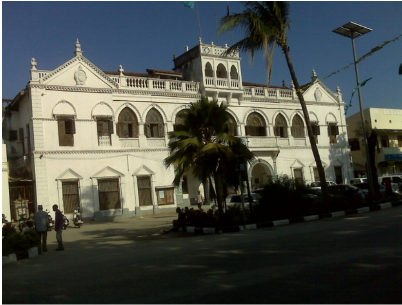
Fig. 10: Front View of Bharmal building (Author)
