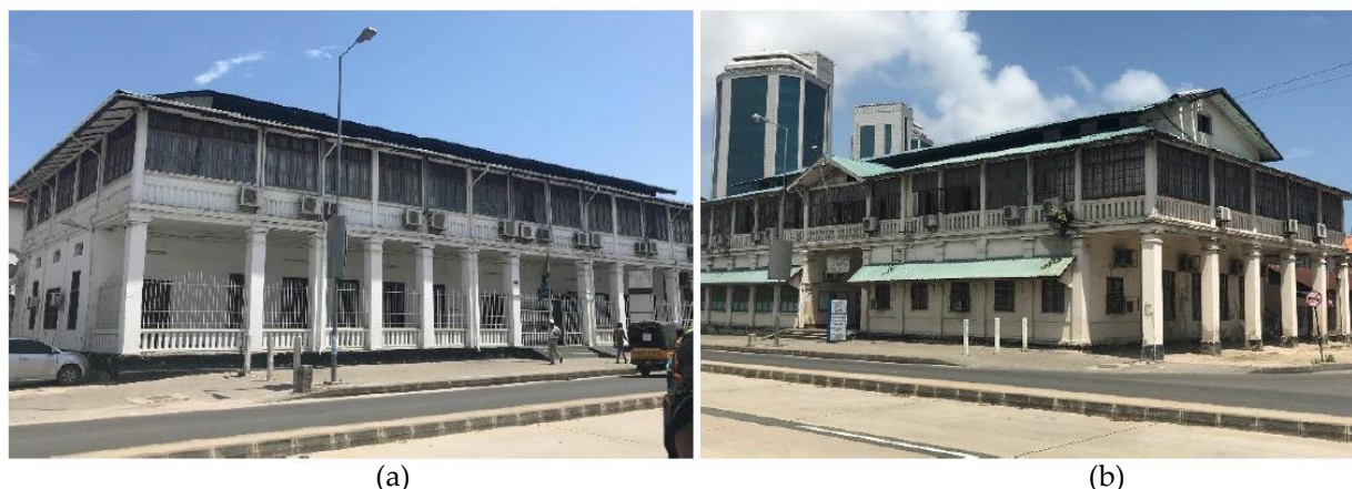
Figure 3. (a) NBS building (b) Survey and Mapping Division building; Series of German buildings with balconies covered to increase the floor plan area. (Source: Author, 2020).
