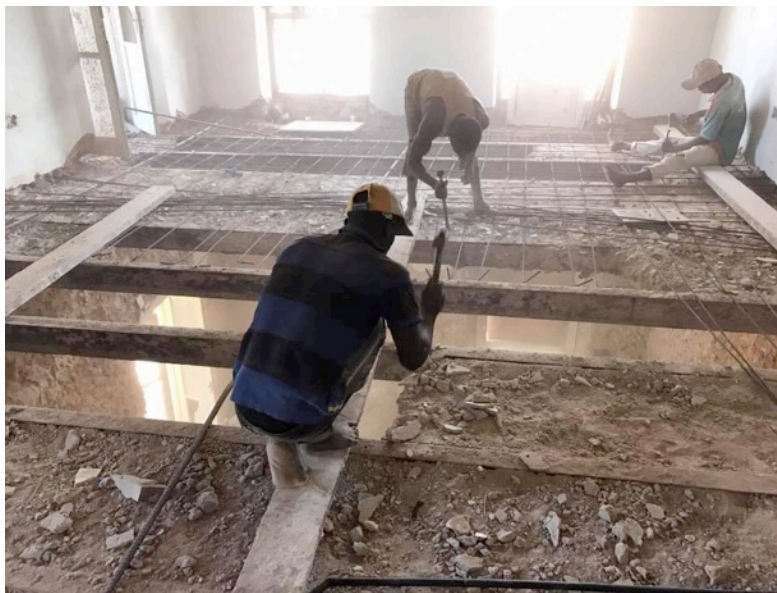
Figure 2: Replacement of structural floor slab during renovations (Courtesy of Abuu Shani).
