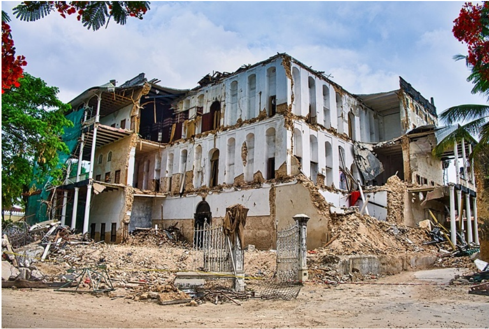
Figure 5: The House of Wonders after 2021 collapses (Courtesy of Abuu Shani).
